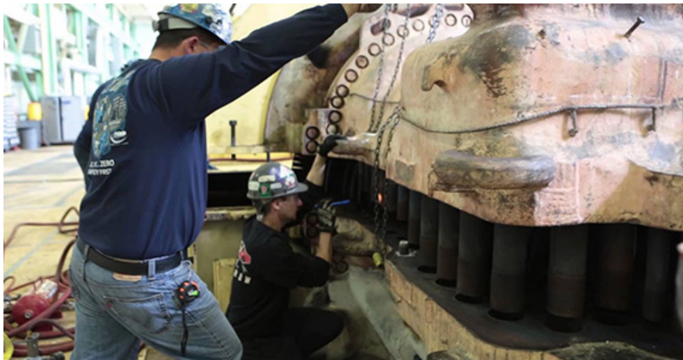
Maintenance workers inspect a turbine. | Turbine Generator Maintenance
