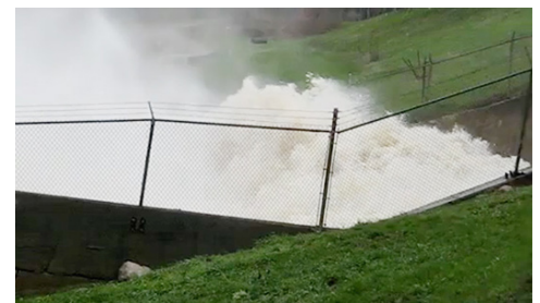
Edenville Dam spillway
